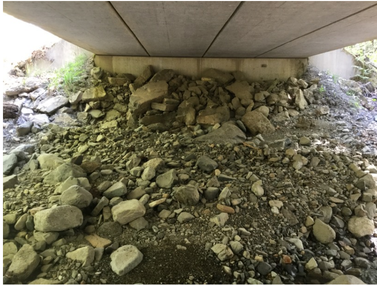
Left Bank Abutment when facing downstream
