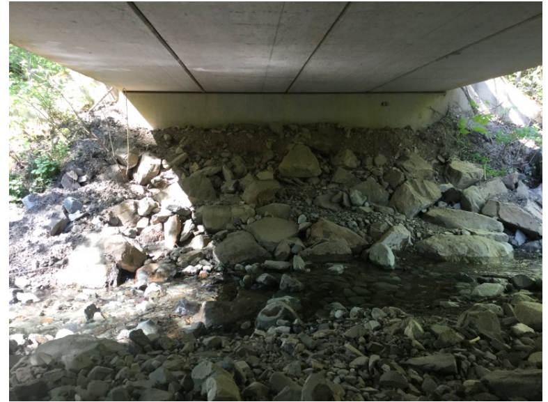
Right Bank Abutment when facing downstream
